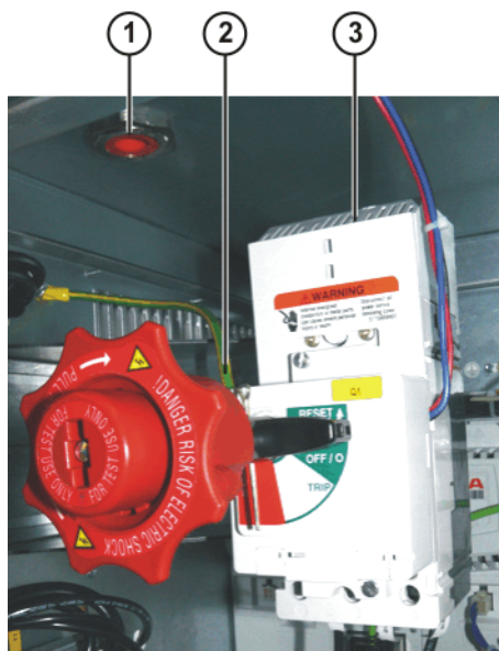
Fig. 6-5: Power supply connection at main switch
